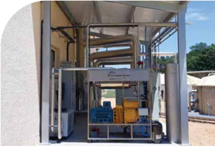
Two Capstone C65 microturbines produce electricity and thermal energy from biogas generated on-site during the treatment process.
